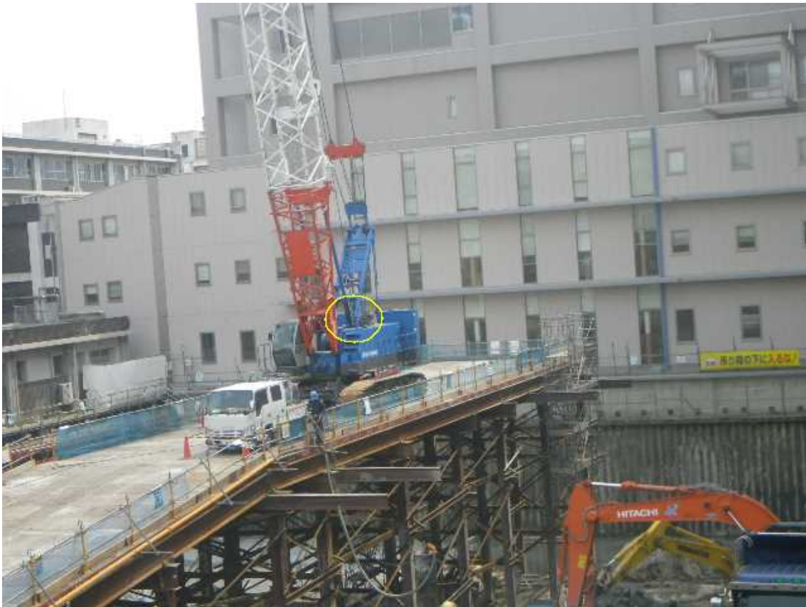
At a hospital construction site.
